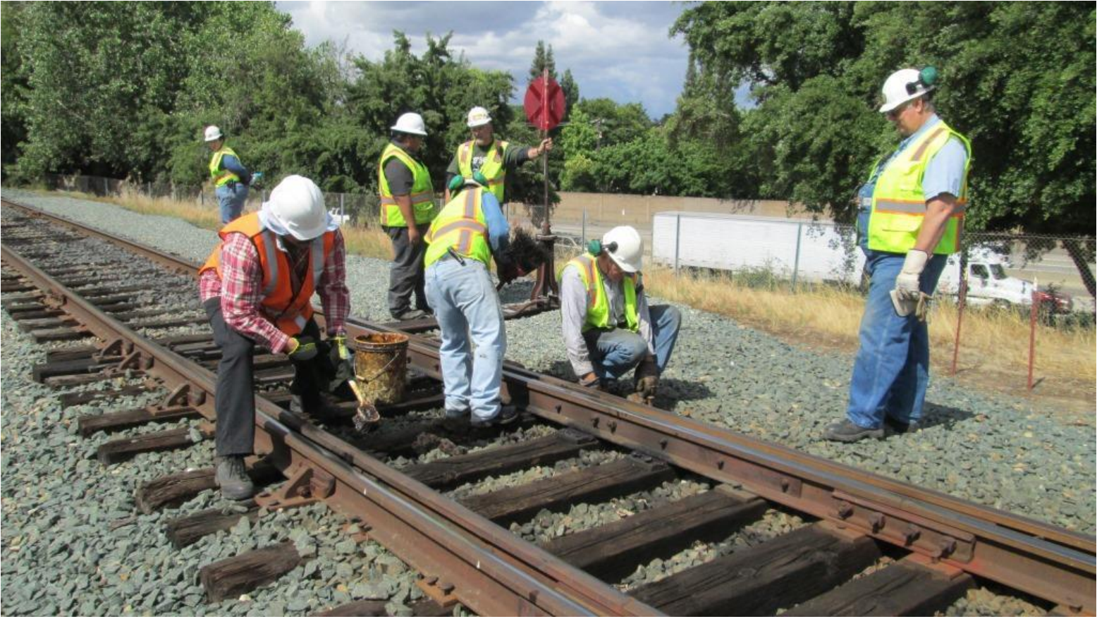
Lookout Heather looks out for the rest of the Team servicing Switch 17
