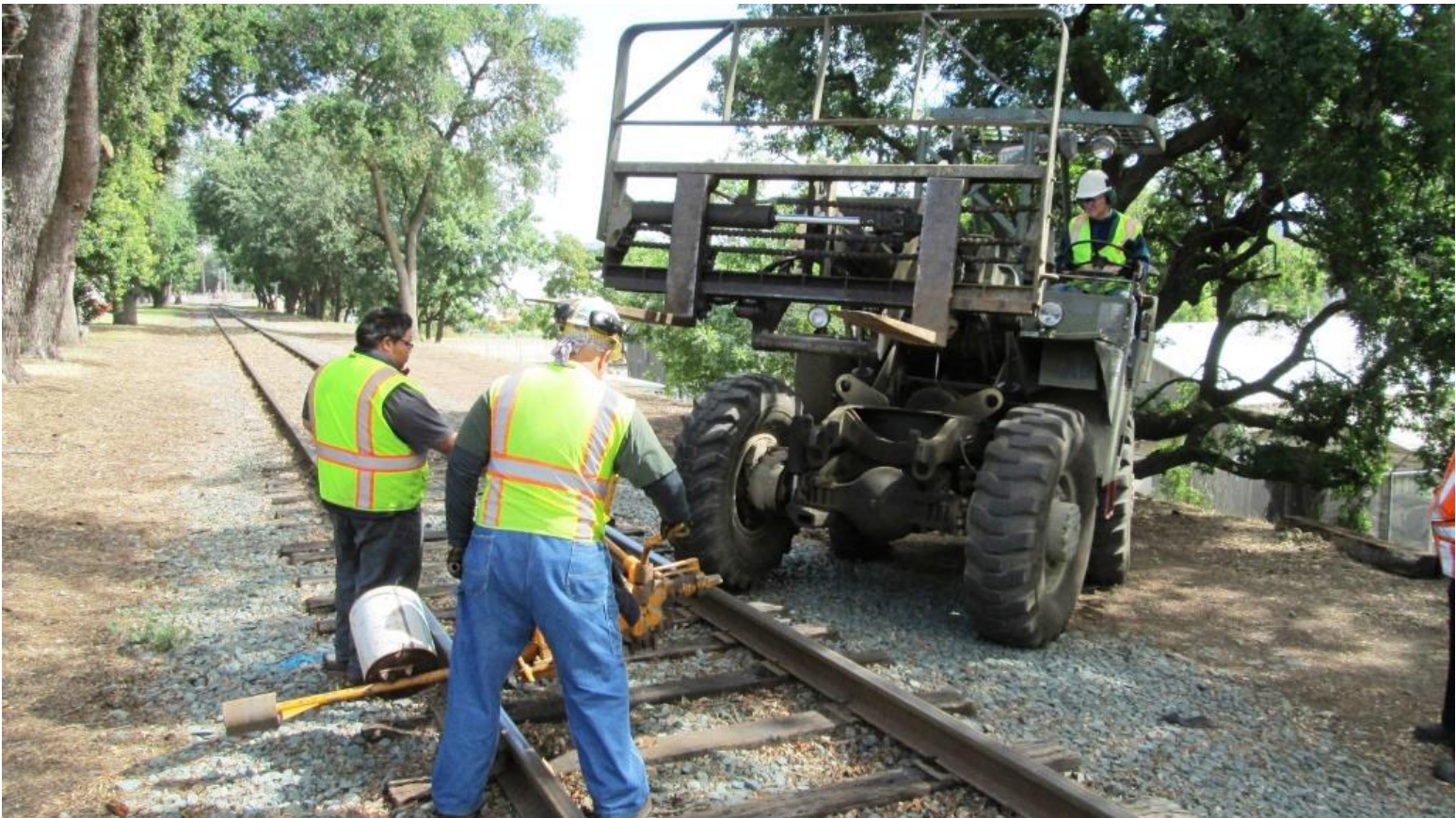
Steve on Big Green grabs the yellow bolt machine and, with Anthony and Mike F.'s help, spin it around to tighten bolts on the east rail
