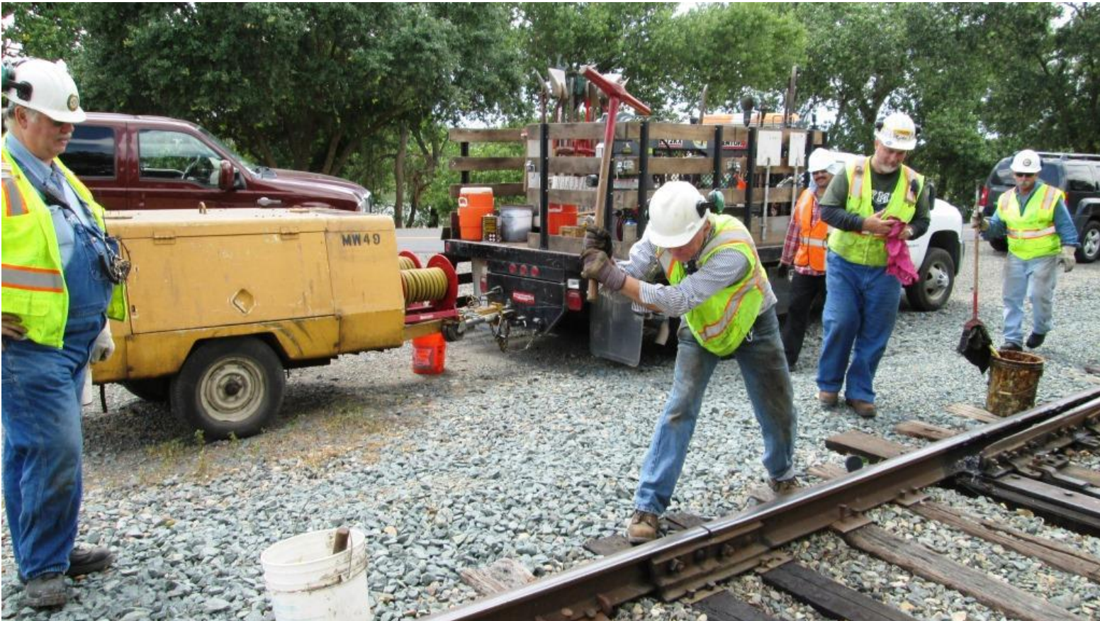
Steve demonstrates his world famous as seen on TV windmill spiking technique on a couple of spikes at Switch 20
