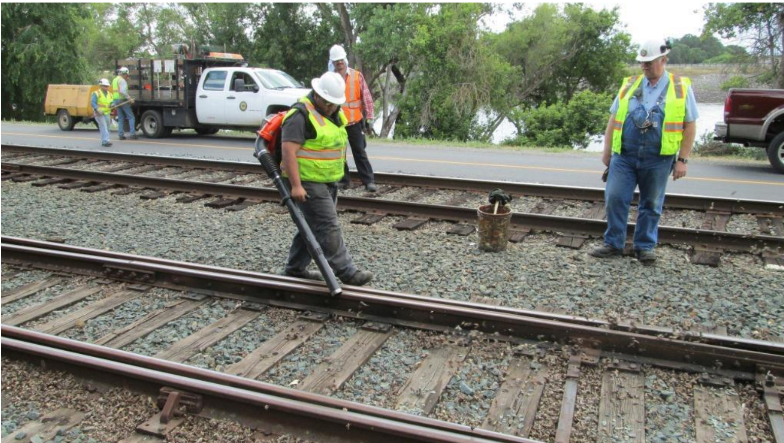
Anthony with the "huff-'n'-puff" machine clears organic debris from between the switch-points
