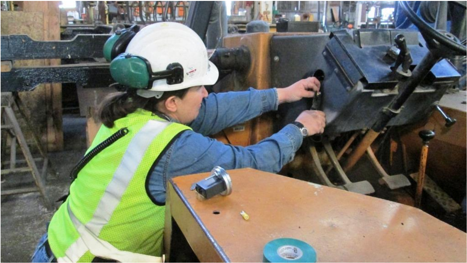
Heather installing a new hour-meter on the back-hoe
