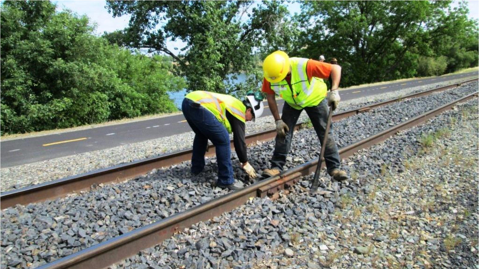
With joints clear of debris further south, Chris M. joins Pam up north to help clear away rock from around the bolts
