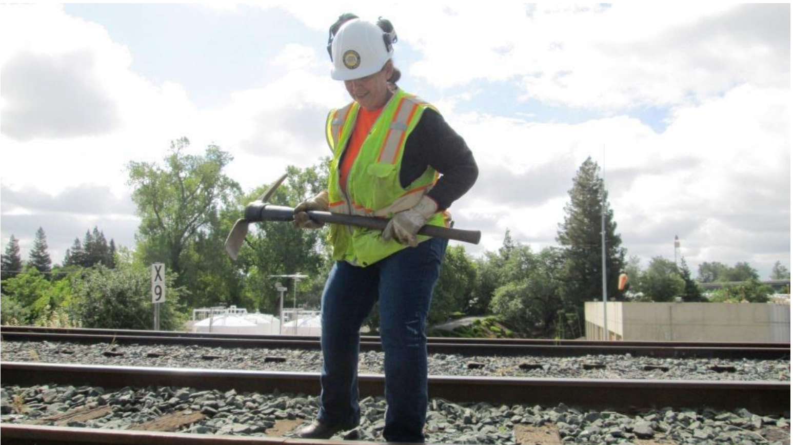
Pam clears away ballast-rock from around joints so that it won't interfere with the bolt-machine
