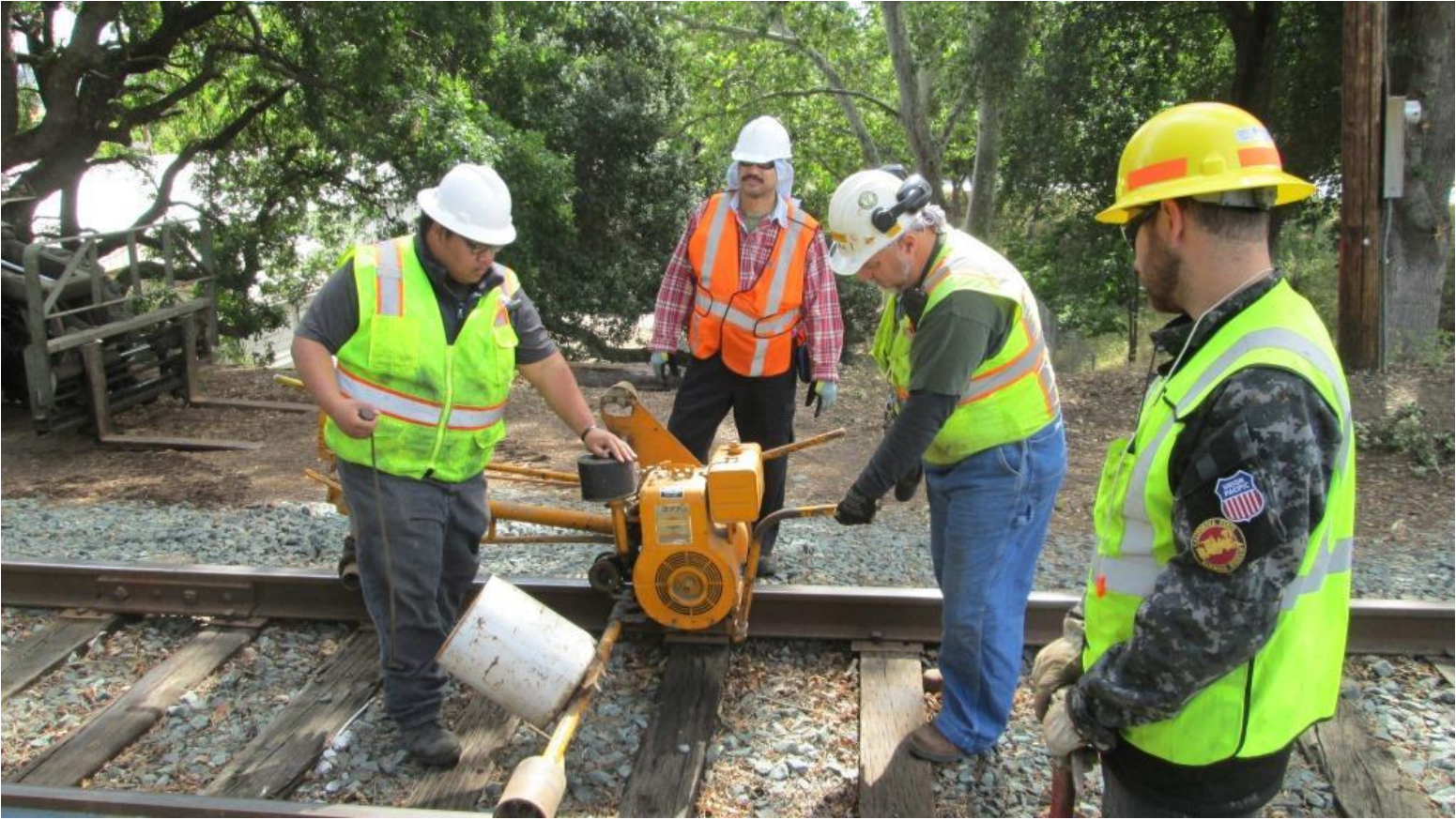
Anthony yanks on the pull-start. Mike F. and Jose get the machine moving. Chris M. stands by with the mattocks to clear debris at joints
