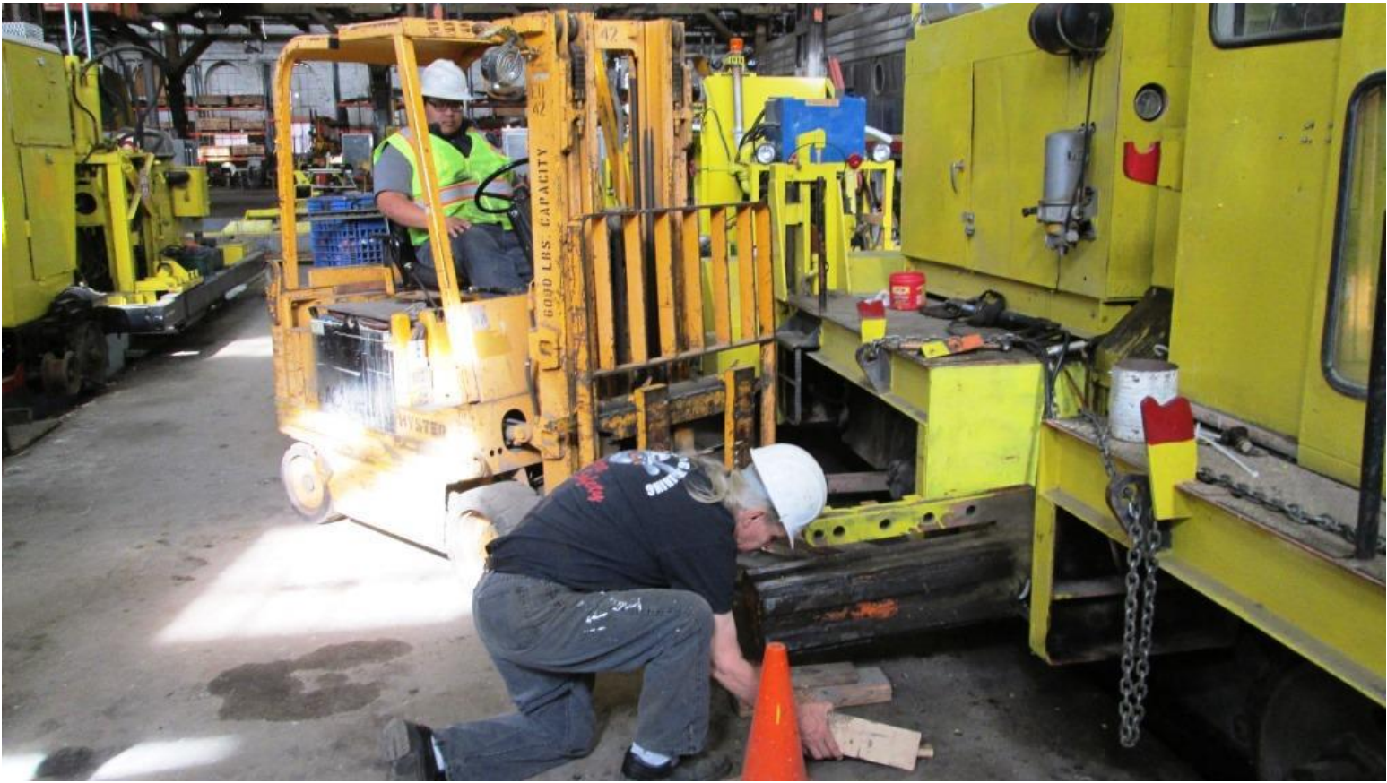
Anthony on the forklift holds the pivot-arm up as Fred places cribbing beneath it
