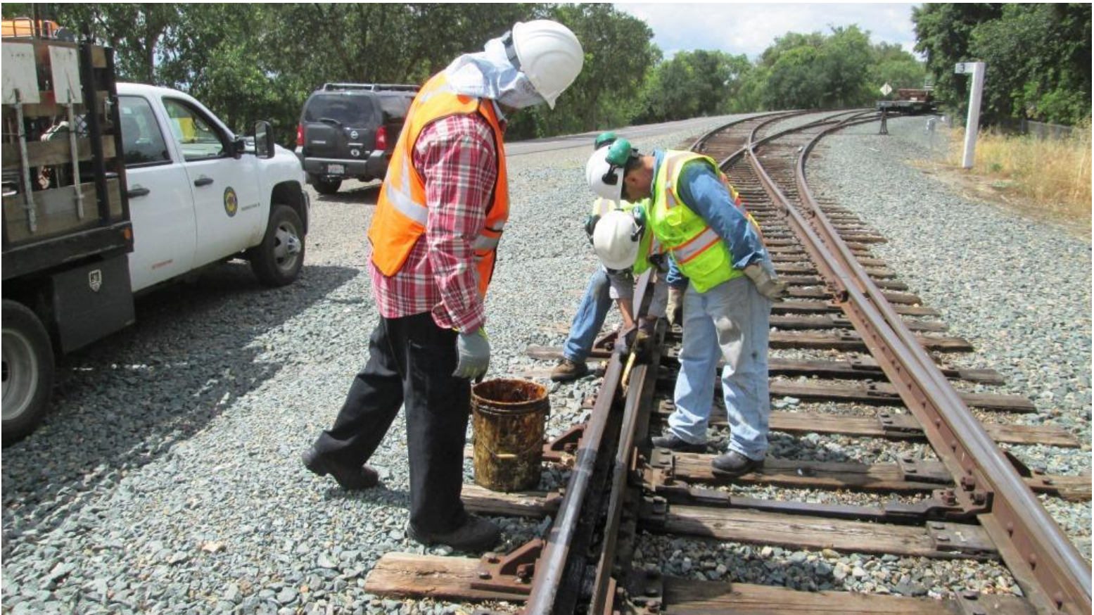
Steve demonstrates proper switch-grease application protocols
