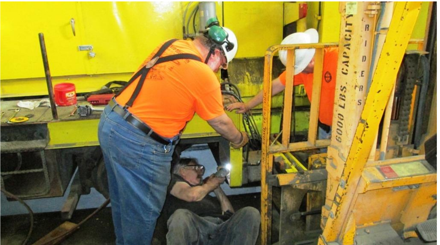
With the head of the bolt severed, Fred works under the machine to remove the rest of it
